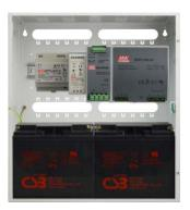
• MEAN WELL built-in power supplies of the following series: RS-xxxx + PSDIN1 / PSDIN2
